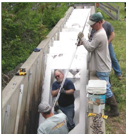
Thames Valley TU members installing new aluminum baffles in the Versailles Pond fishway.
